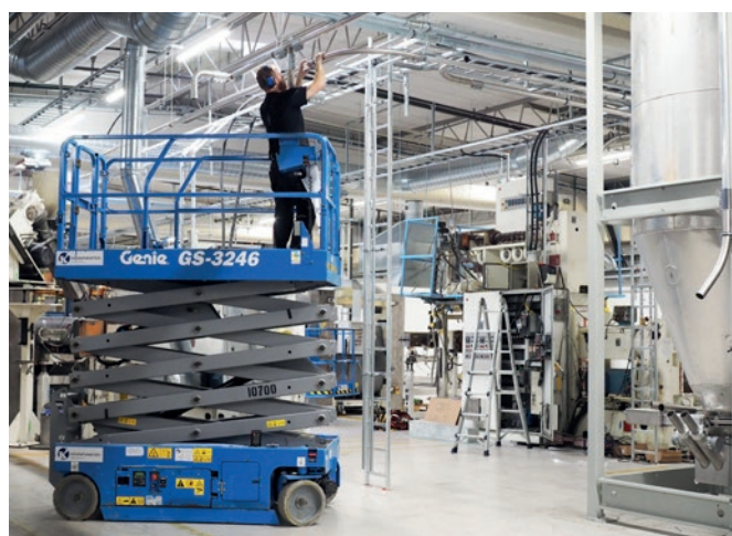
When installing one of the new machines at Scanfill.
